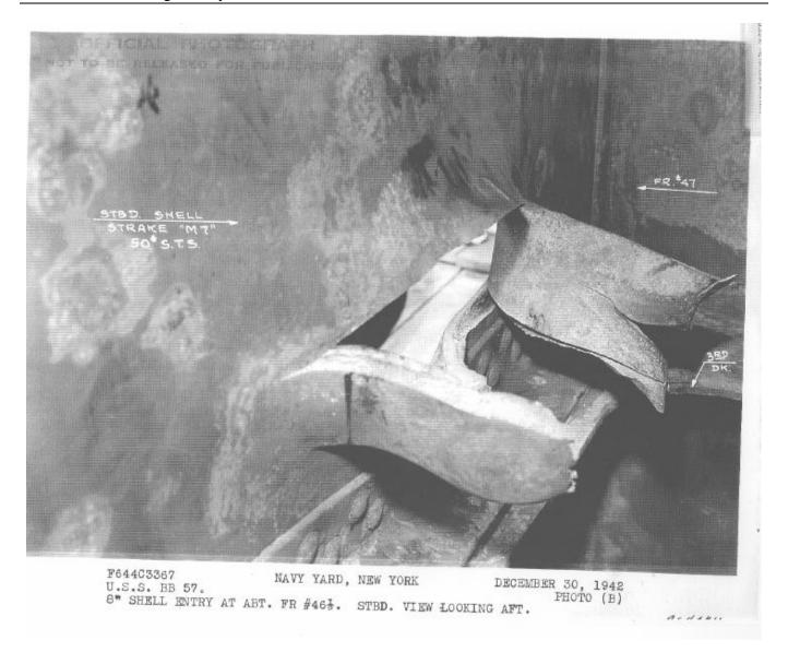
Figure 12 – Hit 4 – Inside view of Entry Hole
