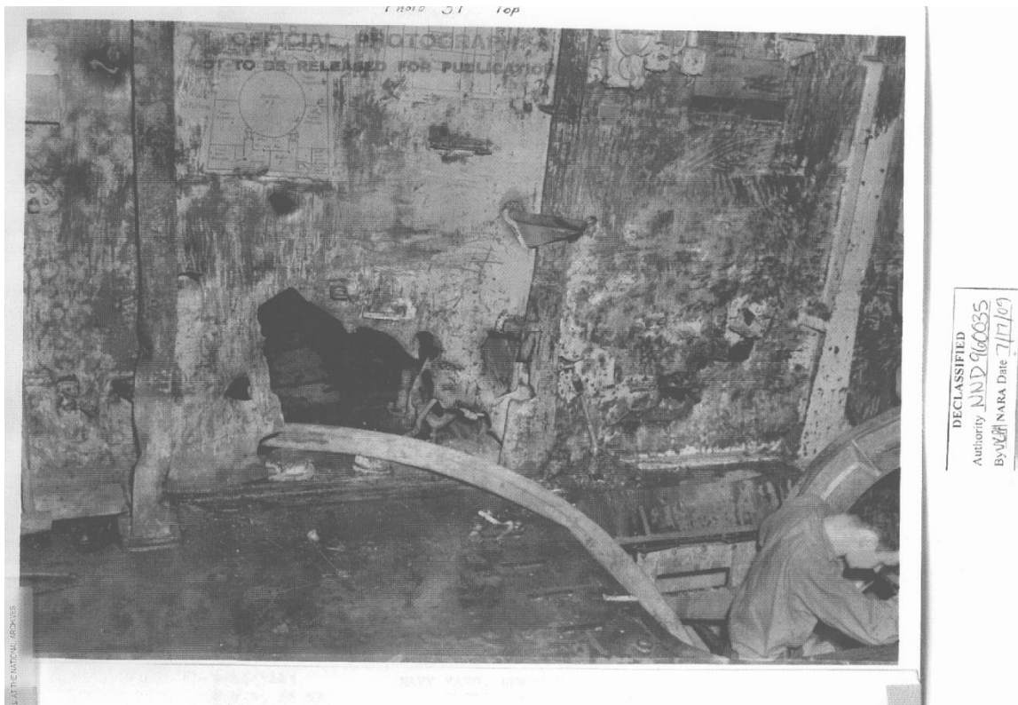
Figure 97 – Hit 26 – Damage to Bulkhead 129
