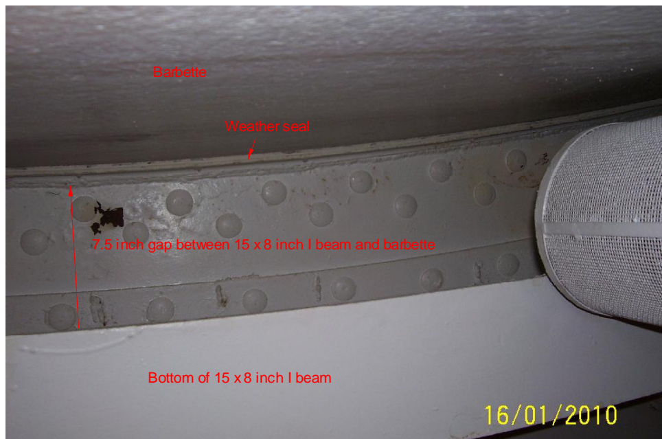
Figure 95 – Hit 26 – Circular I-beam and Barbette on USS Alabama Photograph of USS Alabama copyrighted by Robert Lundgren
