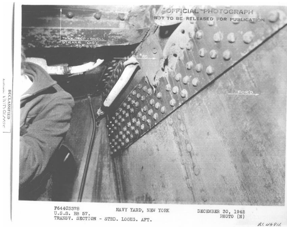
Figure 71 – Hit 20 – Interior Damage to Transverse Section
