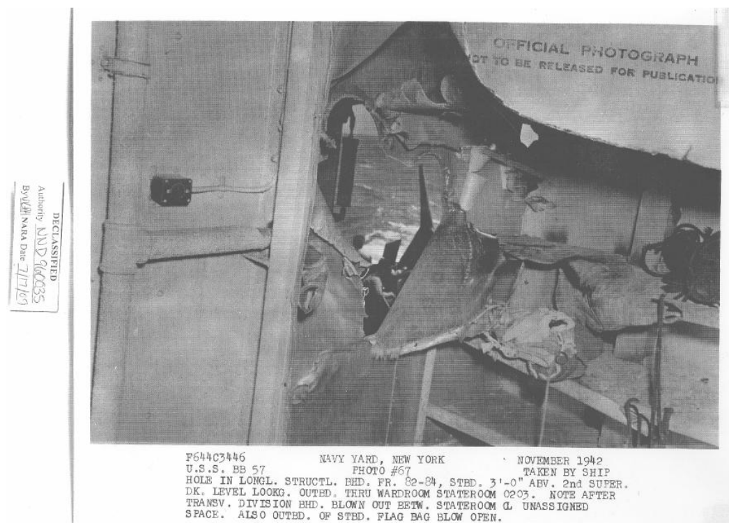
Figure 55 – Hit 17 – Reverse View of Entry Hole
