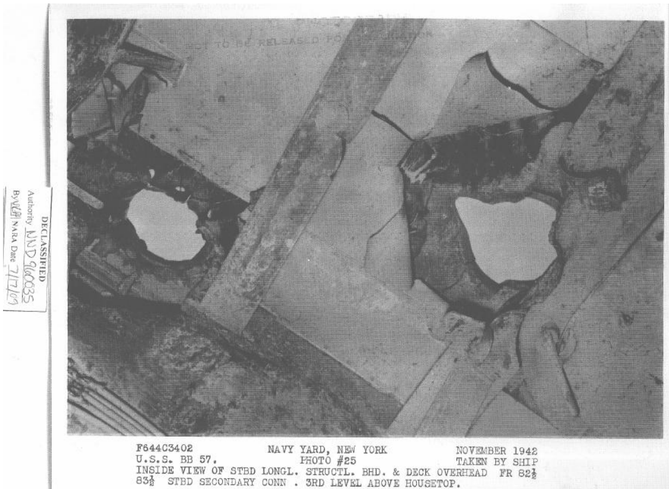
Figure 44 – Hits 14 and 15 – Reverse view of Entry Holes
