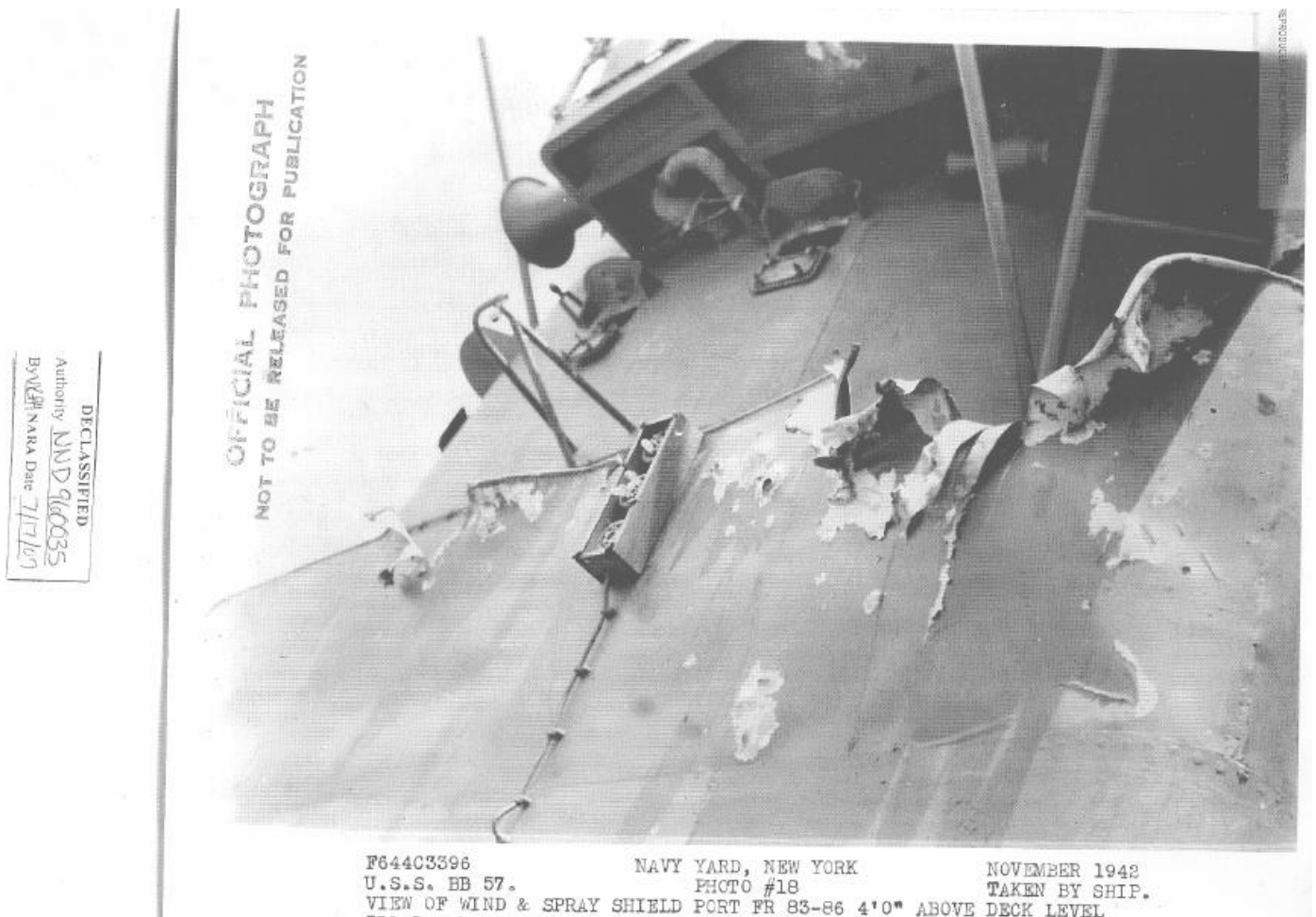
Figure 52 – Hits 13, 14 and 15 – Exit Holes – View C
