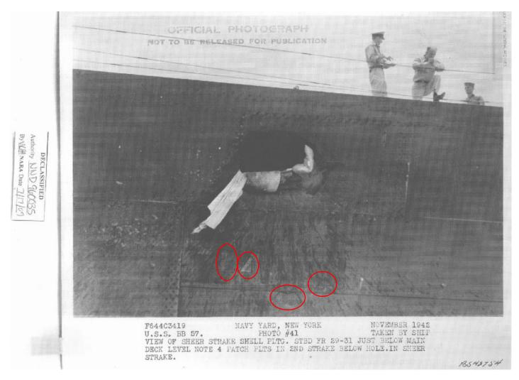
Figure 8 – Hit 2 – Starboard Bow at Frame 30
